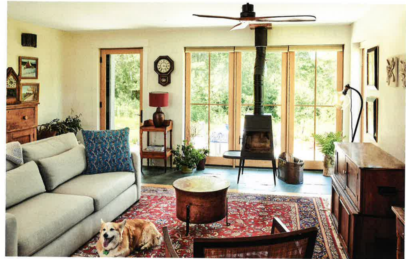
Tall windows are instrumental in connecting indoor and outdoor spaces. The architect specified double-pane windows but has since started using triple-pane units for added performance.
